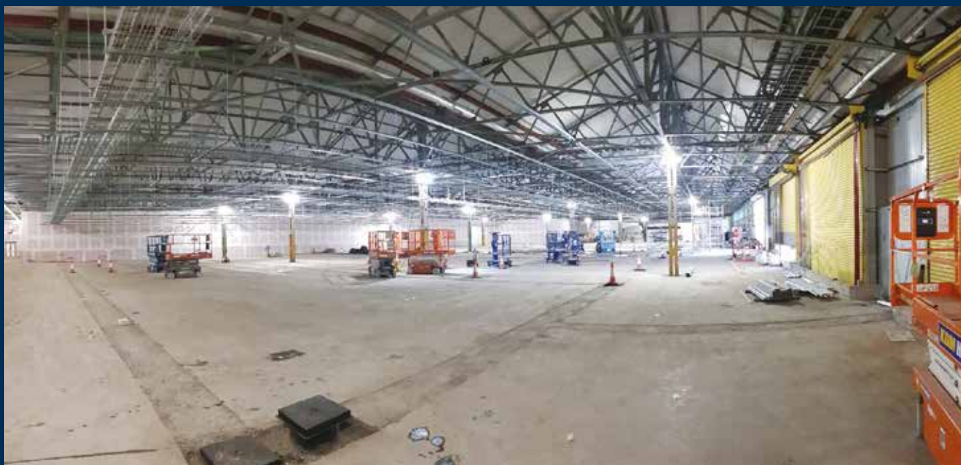
Figure 3(7): Main hangar space immediately pre-pandemic – which was quickly converted to provide laboratory, logistic and engineering capabilities
